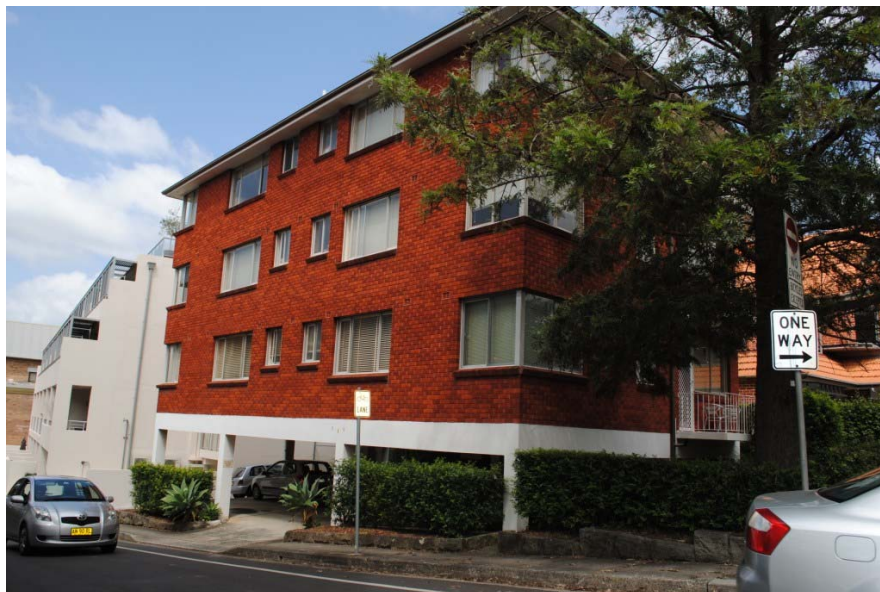
Figure 4: 5 Mandolong Road looking west showing elevation to Melaleuca Lane
