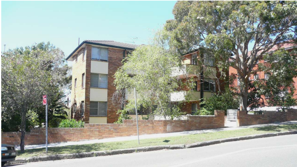
Photograph 3: The adjacent residential development on the opposite side of Melaleuca Lane.
