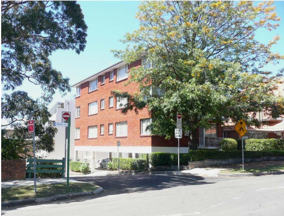
Photograph 1: The site and the existing building on the corner of Melaleuca Lane.
