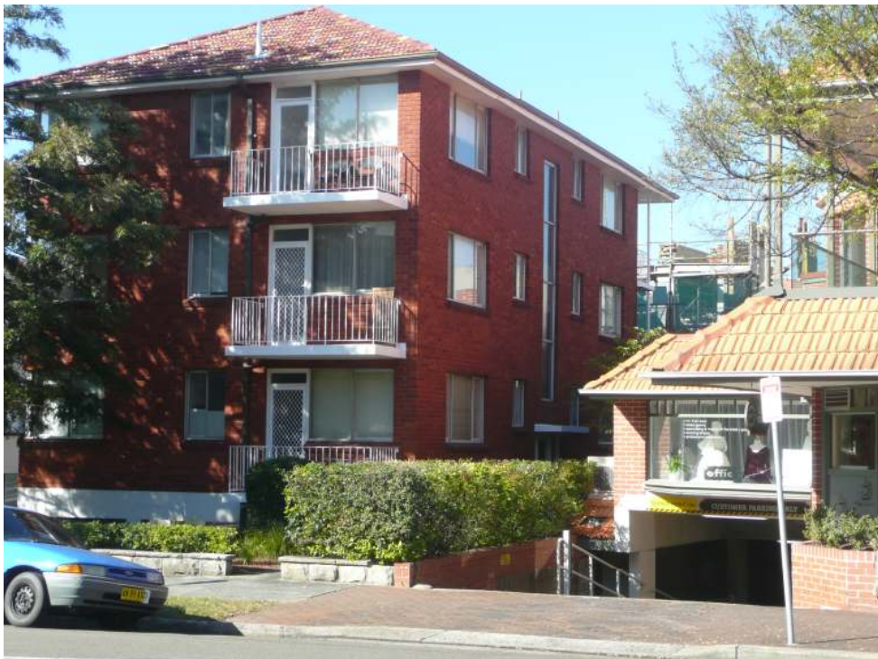
Photograph 2: The site and existing building viewed from Mandolong Road.
